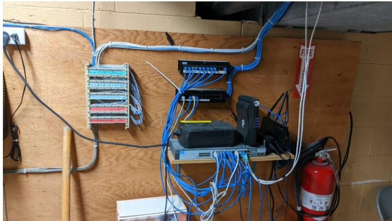
We recommend replacing the existing cable runs entirely, new cables to be run inside walls / above ceilings where possible and installed in raceways if necessary. All cables should be brought back to a single central point. All cables should be labeled clearly at both ends for ease of identification and, at the server end, cables should terminate in a patch panel.
